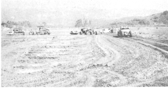
Fig. 1. Beginning construction of the reservoir.
