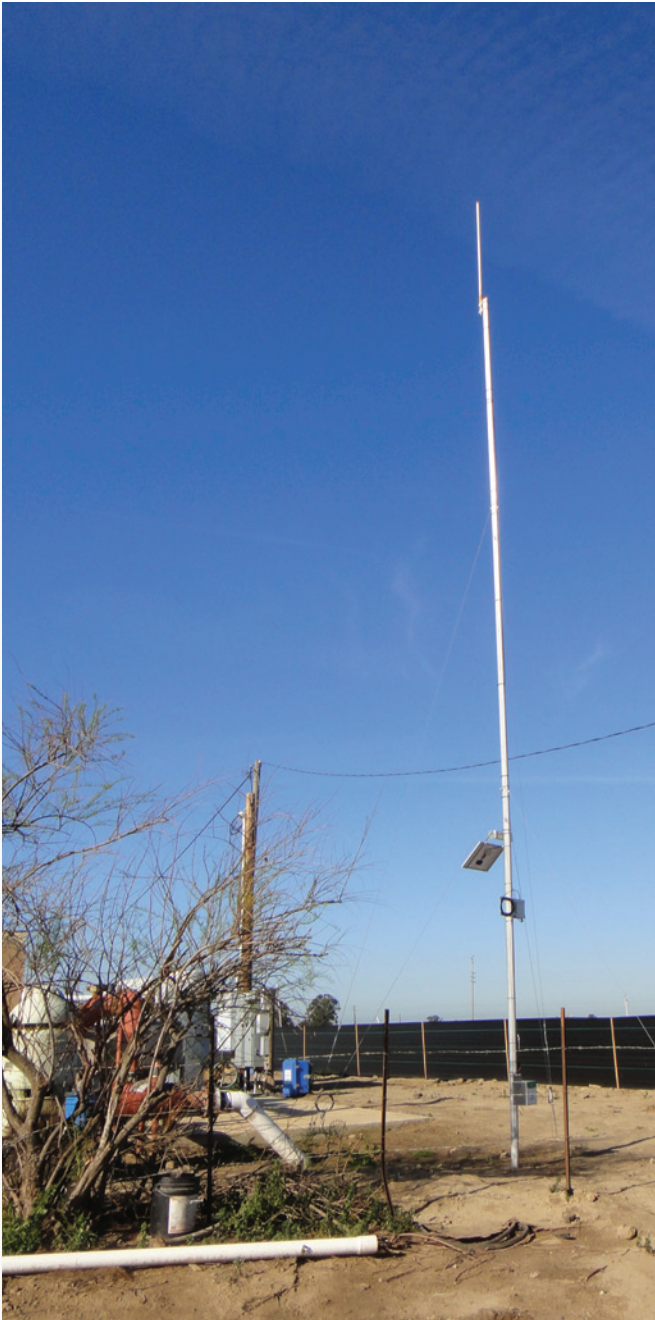
Figure 7. Weather stations can be equipped to measure solar radiation, wind speed, rainfall, relative humidity and temperature. Some monitoring stations indicate when a problem has occurred with the irrigation system.
