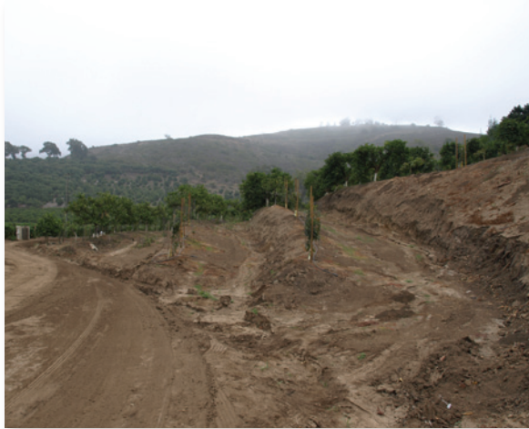
Figure 16. Terracing an avocado orchard with the contour of the hillside will direct water runoff along contours rather directly down the slope which flow direction, slowing runoff and resulting in less erosion. Terraces are angled into the hillside to control the conveyance of water.
