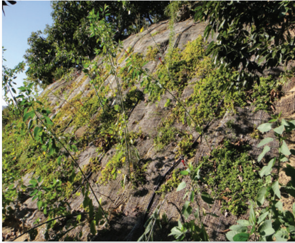
Figure 14. ‘Critical Area Planting’ with jute netting below. Jute netting helps retain the soil on the slope while the plants are becoming established. Once plants are established, the netting is biodegradable and turns into organic matter in the soil.
