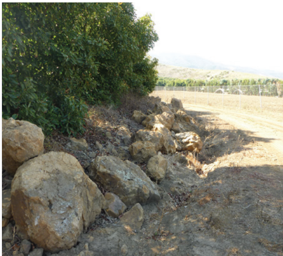
Figure 20. Rock riprap reinforces the toe of the slope helping slow down rain runoff and keeping the soil on the slopes.
