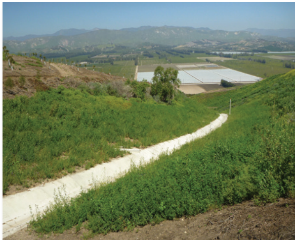
Figure 13. ‘Critical Area Plantings’ consist of single species or a mixture of grasses, legumes, and/or forbs. These plantings provide slope stability and can contribute to plant pest control by following an Integrated Pest Management Program.
