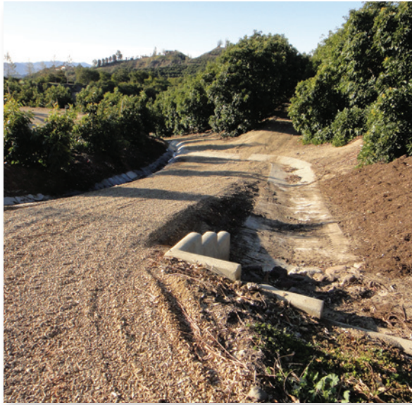
Figure 9. Gravel road reduces dust damage to trees and soil loss through wind and erosion.
