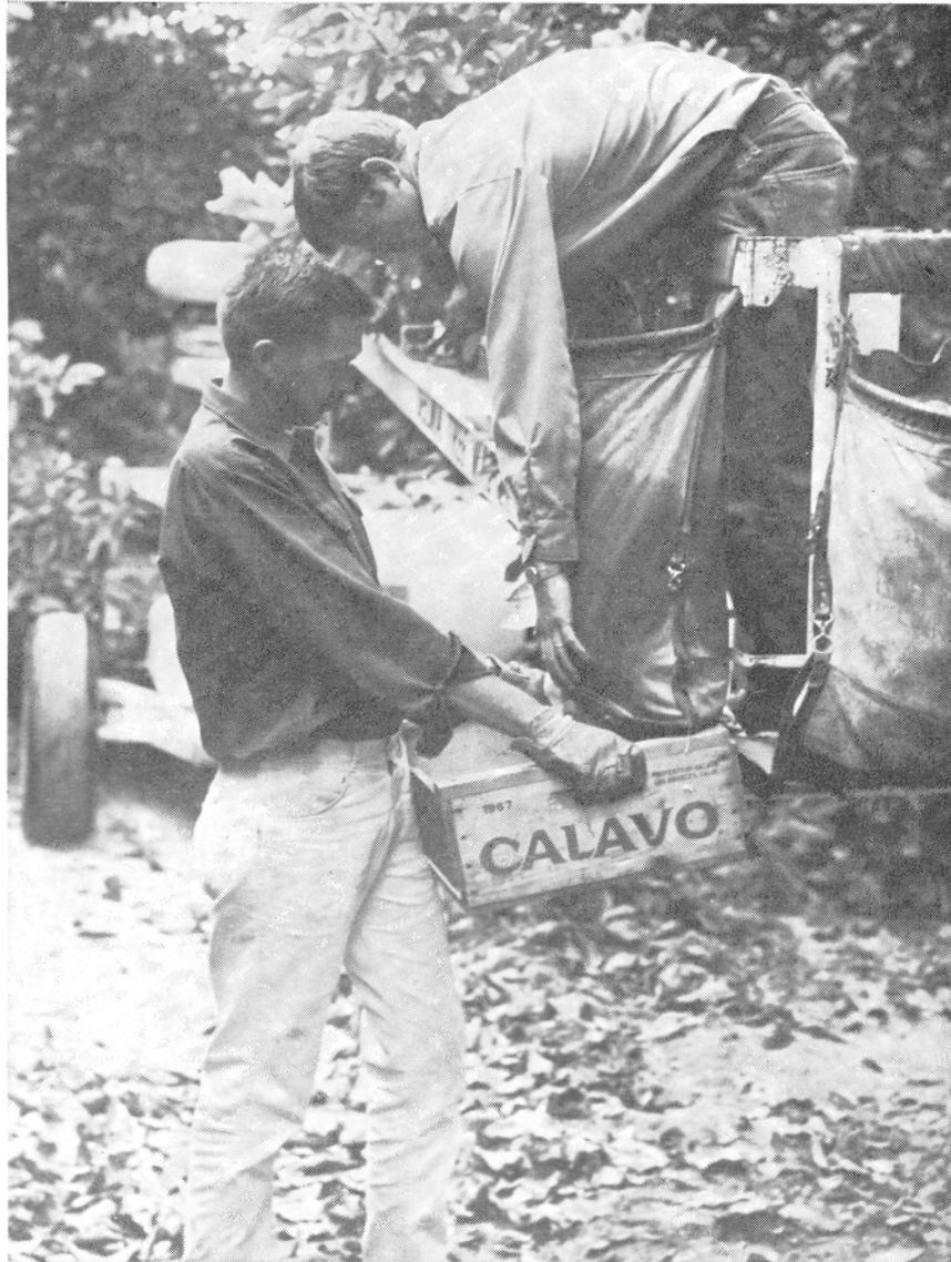
Figure 3—Fruit transfer from picker's work station on machine to field box held by ground assistant.
