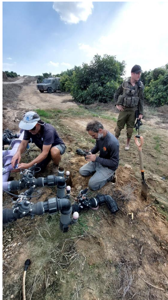
Irrigation controller damaged by mortar bomb is fixed
