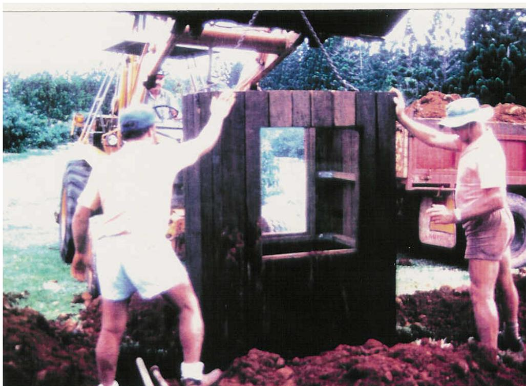
**Fig. 3** Installation of rhizotron boxes constructed for root studies on avocado trees, Maleny, S.E. Queensland, Australia.
