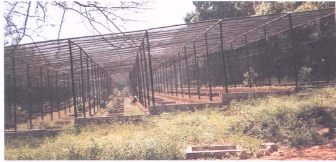
Figure 2 Renovated shade cloth structure
