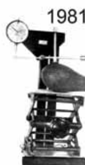
Blackie Swart constructed an instrument whereby fruit firmness could be quantified
