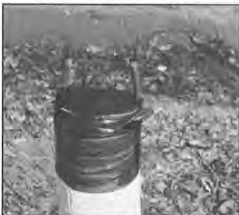
Fig. 28. A black asphalt emulsion seal coats the cut surfaces.
